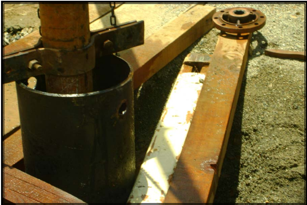
Lowering of Turbine Pump
