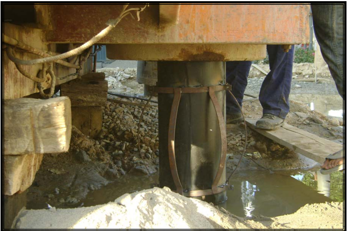
Lowering with Centralizer
