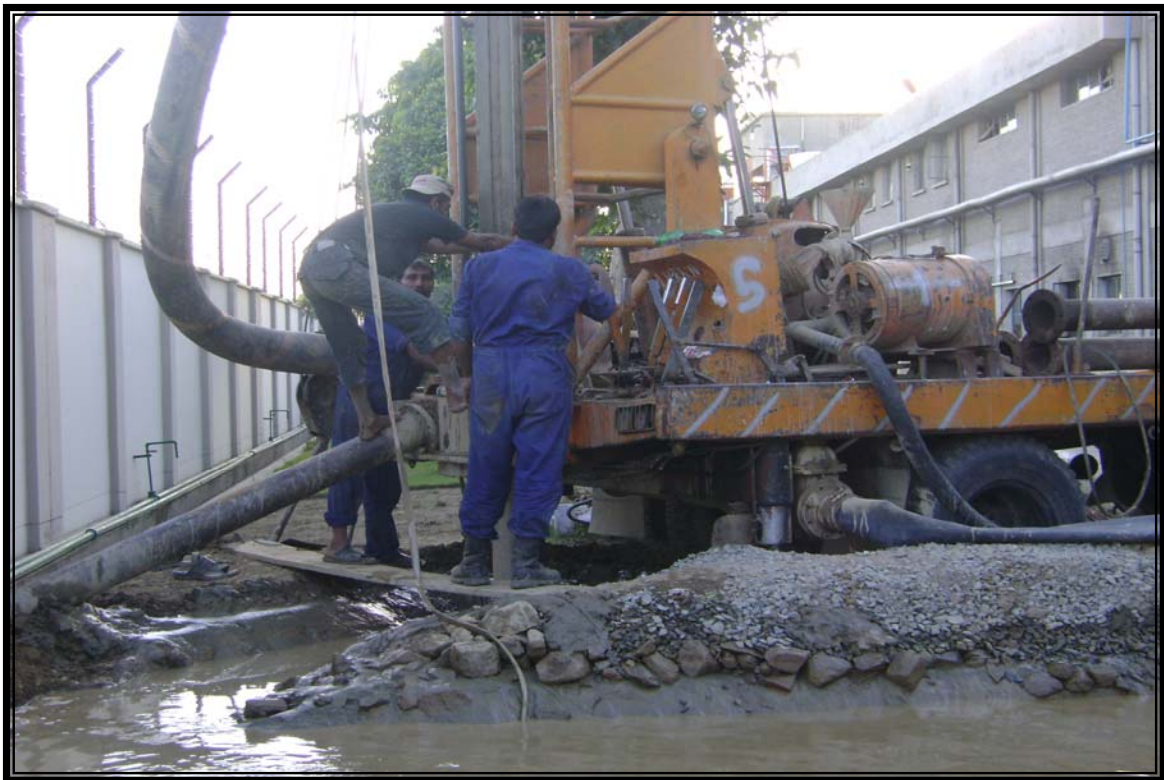
Drilling in Operation
