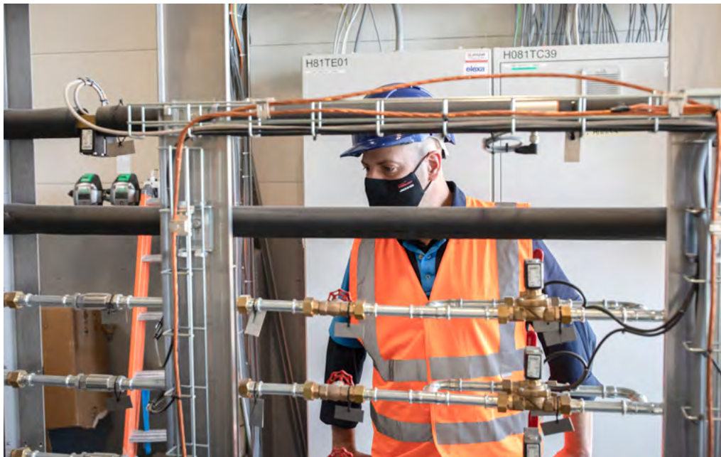
An employee standing next to a pyrolysis machine in our manufacturing facility in Neuchâtel, Switzerland
